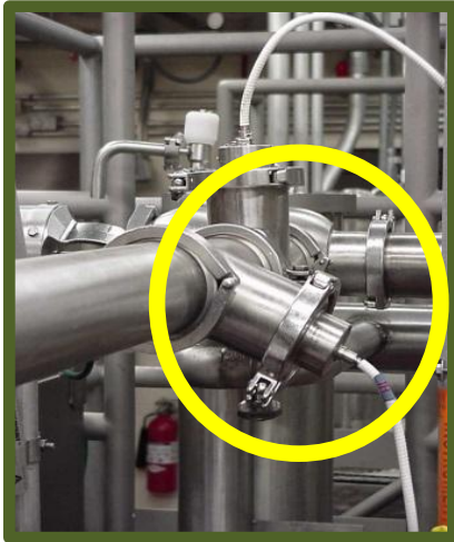
Figure 23. Accumulation/niche created by reassembling the probe facing down instead of
